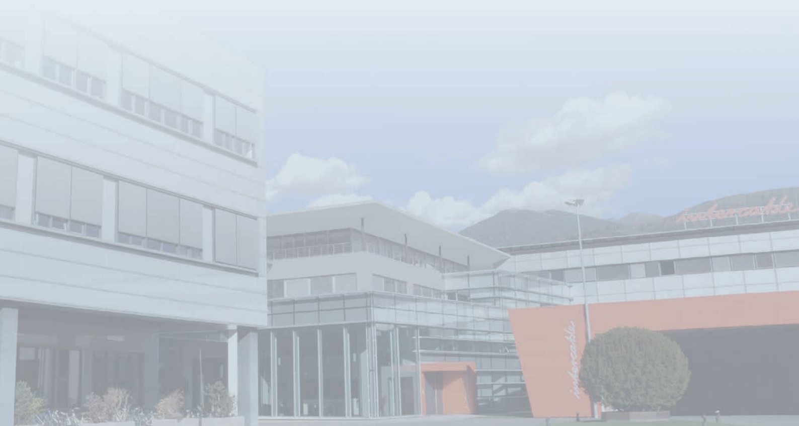
Abb. 5: Intercable GmbH, Headquarter Bruneck
