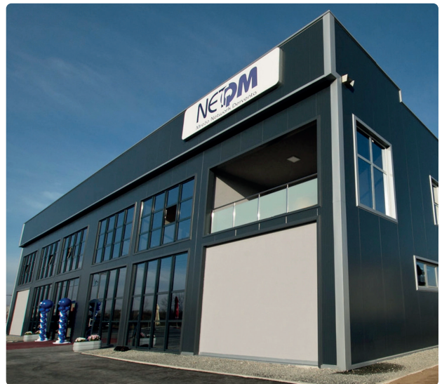
NetQM, production site in Bosnia and Herzegovina
